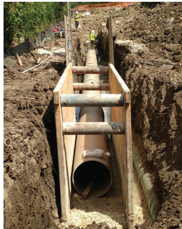
Wastewater line maintenance
