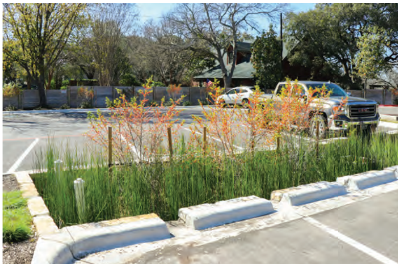
The Ruby Hotel landscaping feature to manage water runoff and filter pollutants
