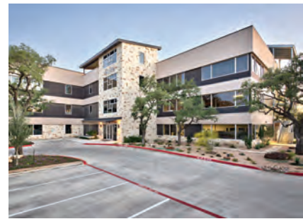
Four Eleven mixed-use building with Class A office space
