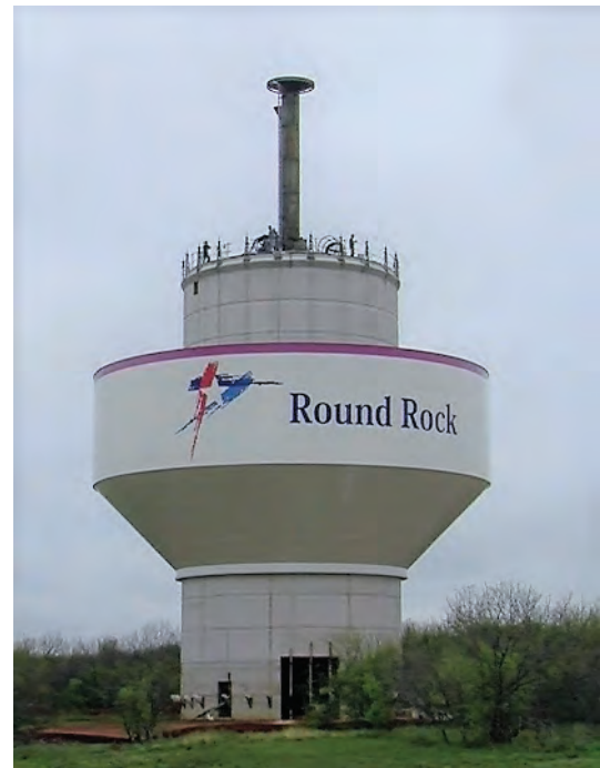
Water reuse tank
