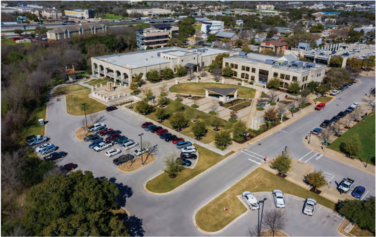
The Allen R. Baca Center, Centennial Plaza, and the McConico building
