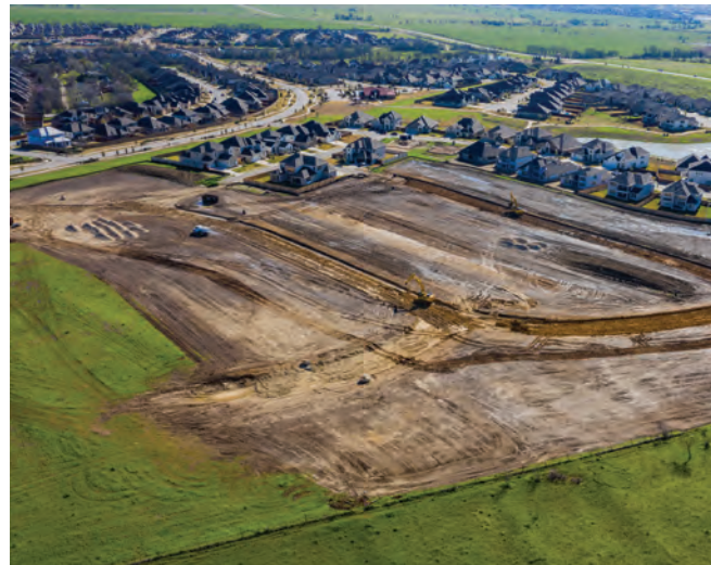
Homes under construction in Round Rock
