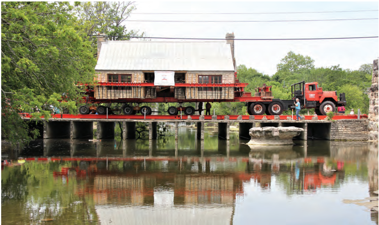
The Stagecoach Inn crossing Brushy Creek before reaching new location at Bathing Beach Park
