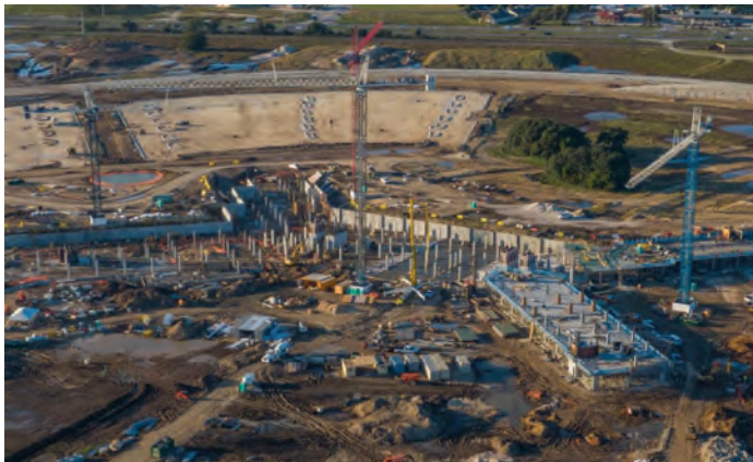
Kalahari Resorts during construction
