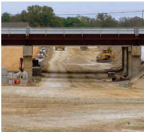
Road under construction
