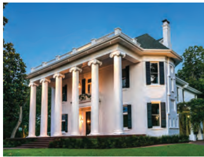
Woodbine Mansion event facility
