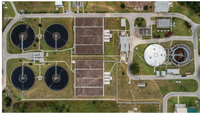
Brushy Creek Regional wastewater treatment plant
