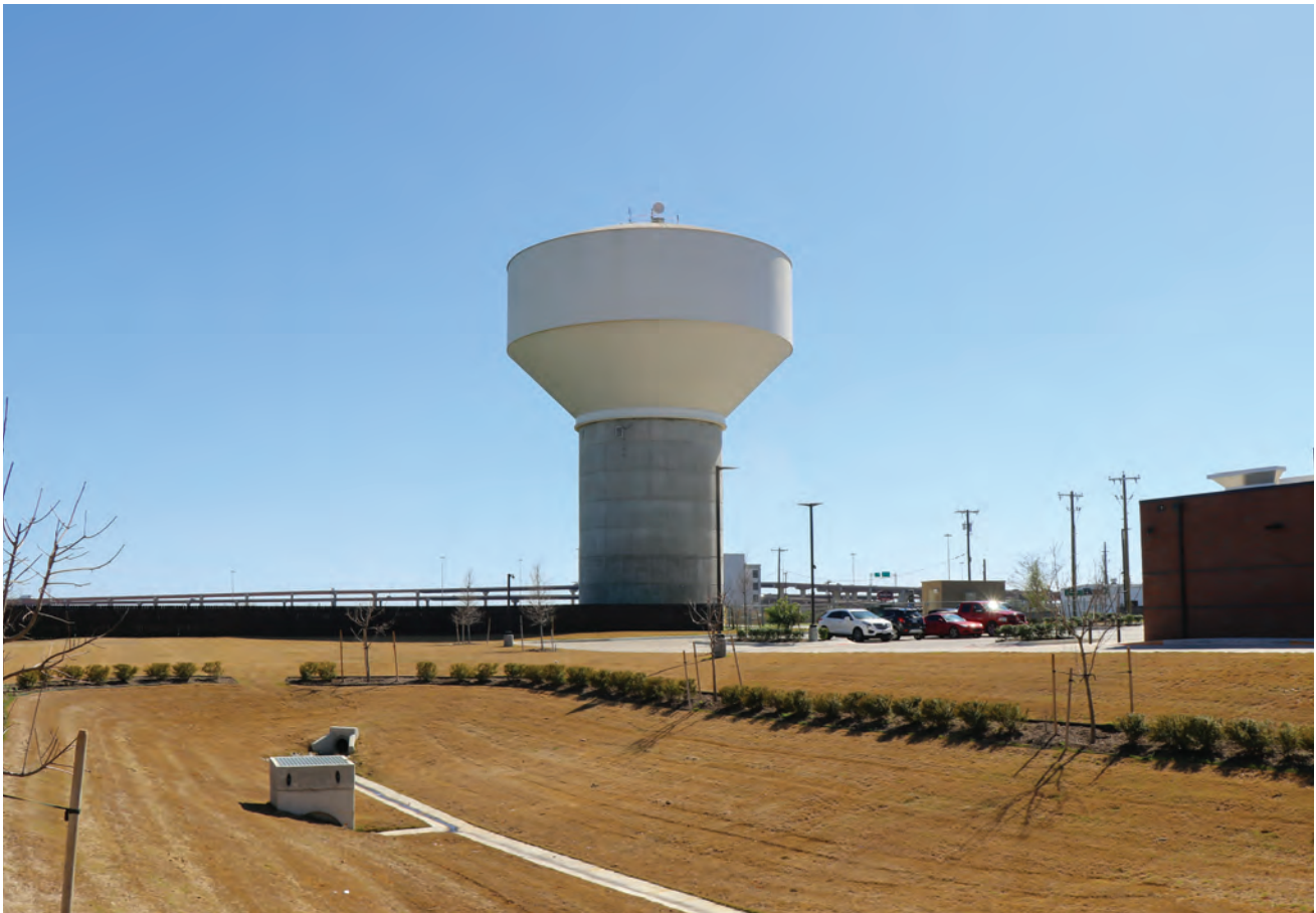
Water tower on Mays Street
