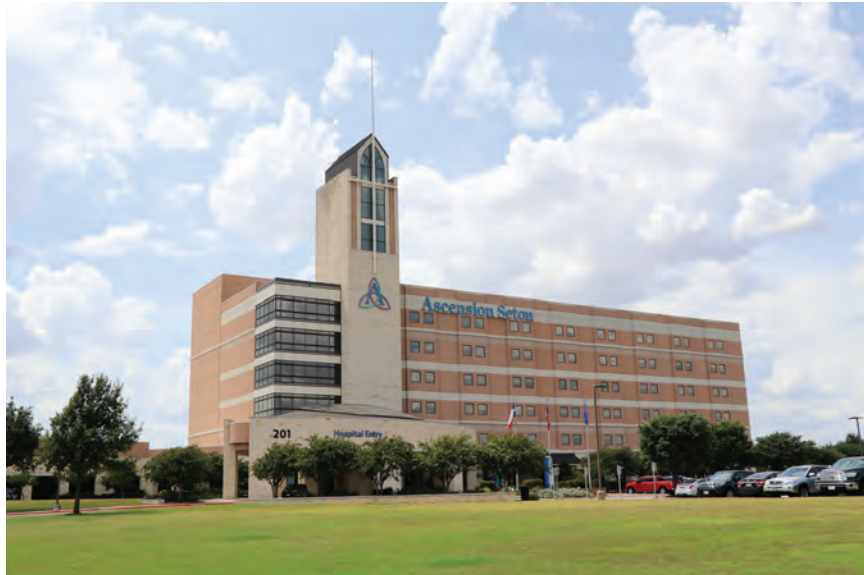
Ascension Seton Hospital in Northeast Round Rock
