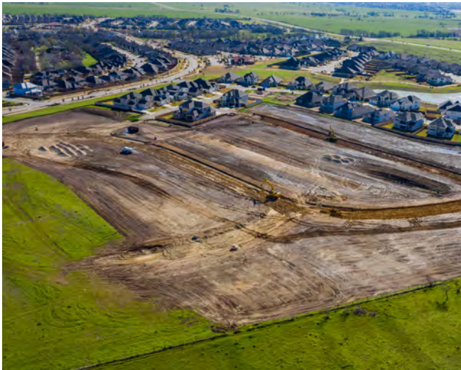
Homes under construction in Round Rock
