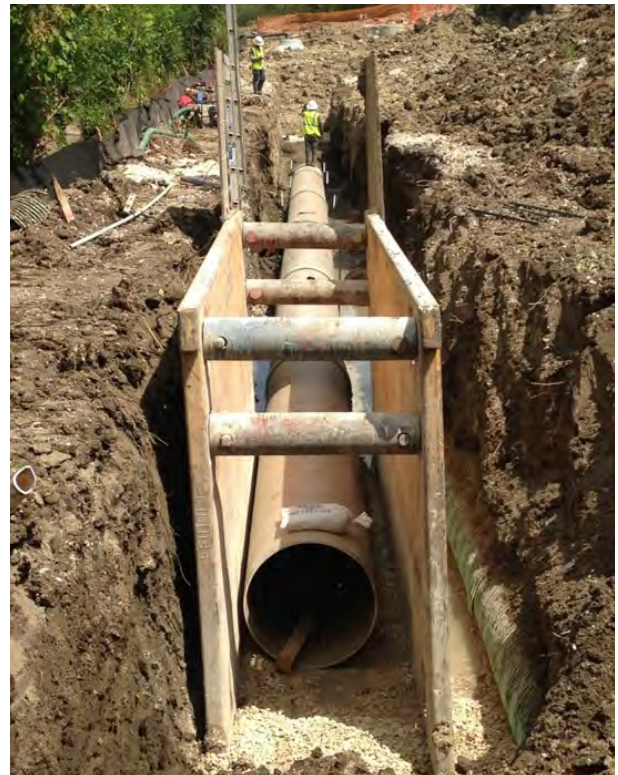
Wastewater line maintenance
