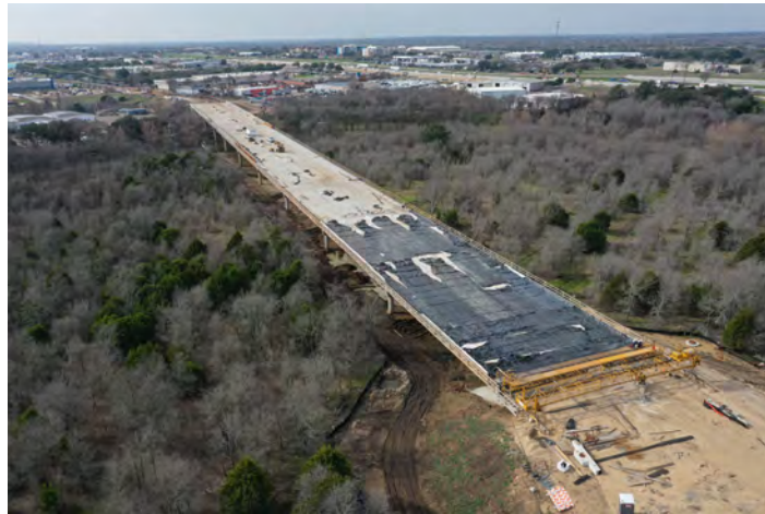
North Mays Street road extension
