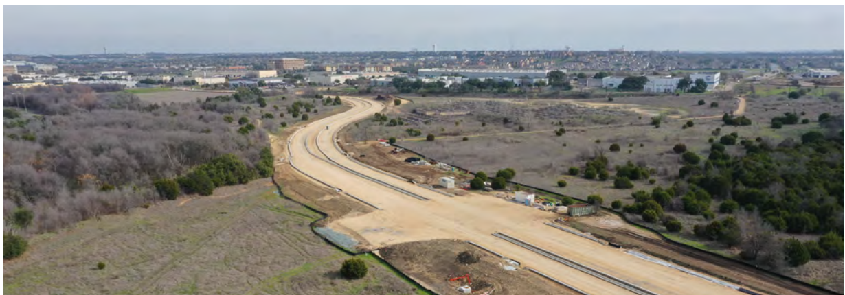
Roadway extension project to improve connectivity
