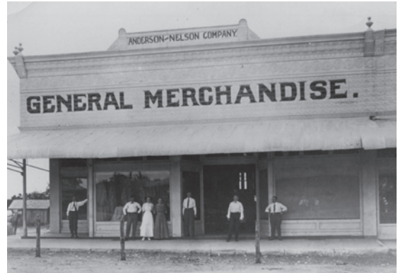
200 E. Main built 1904
