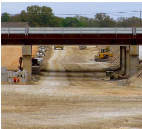
Road under construction
