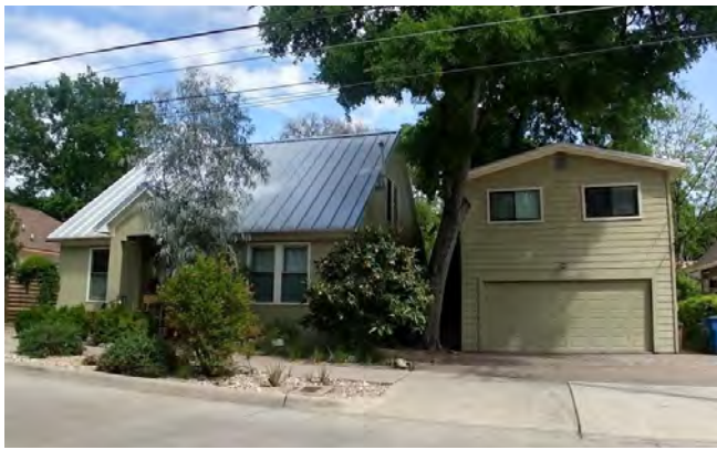
Accessory dwelling unit above garage
