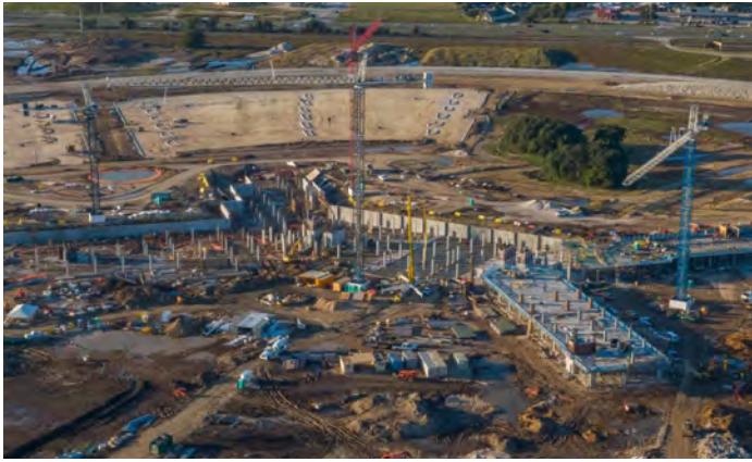
Kalahari Resorts during construction
