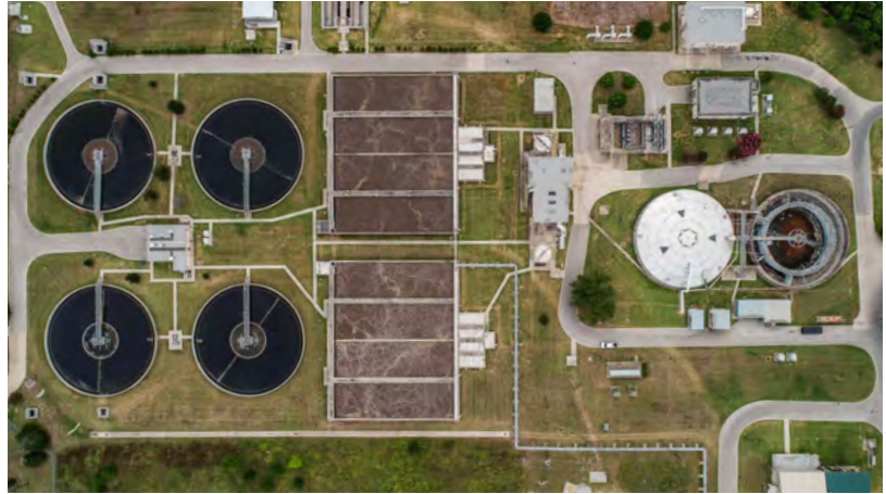
Brushy Creek Regional wastewater treatment plant
