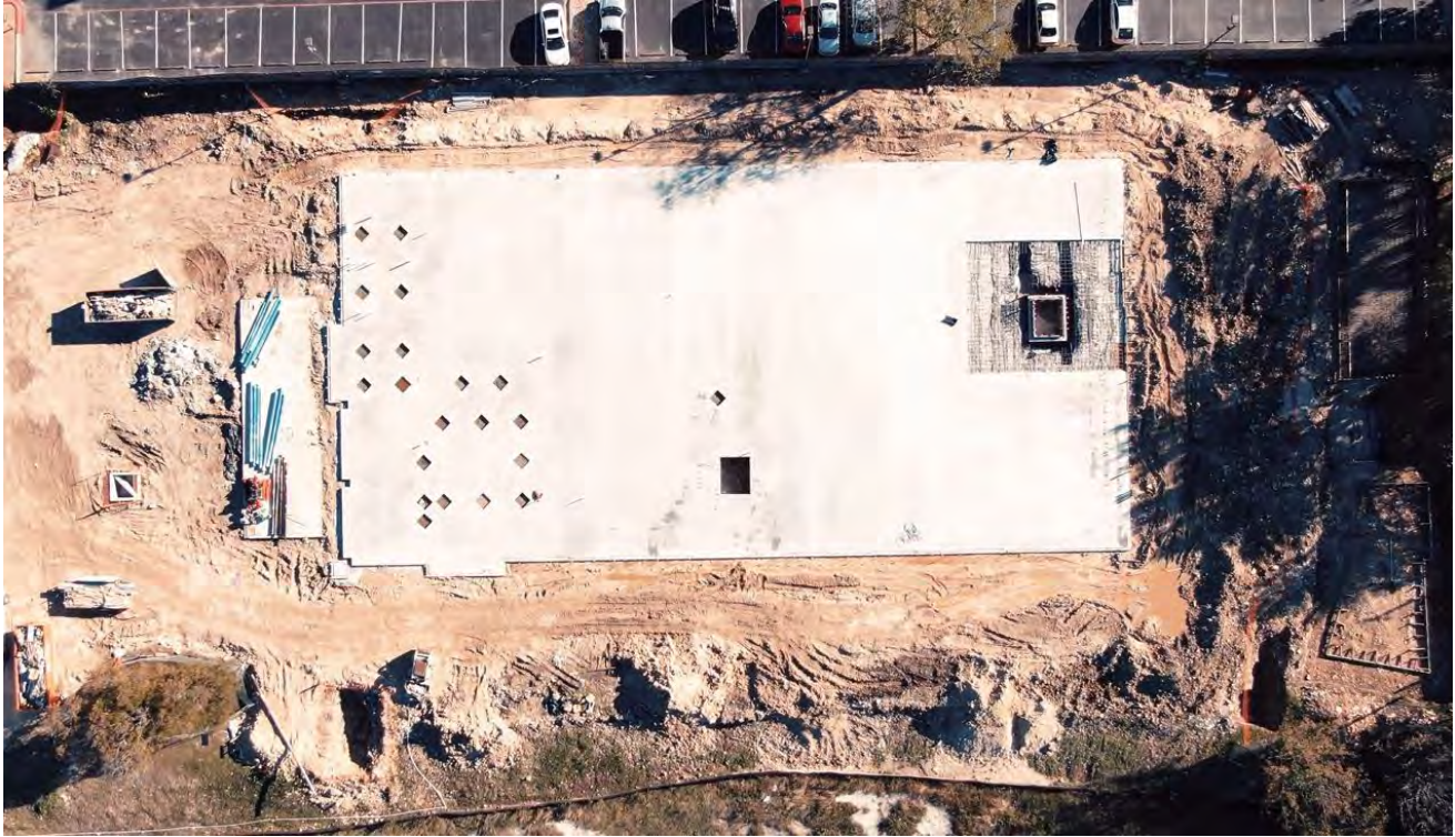
Lot with new construction
