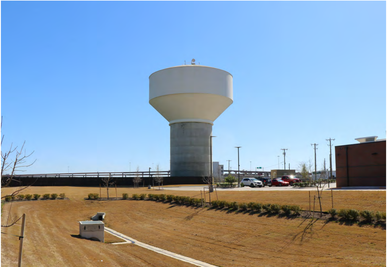
Water tower on Mays Street
